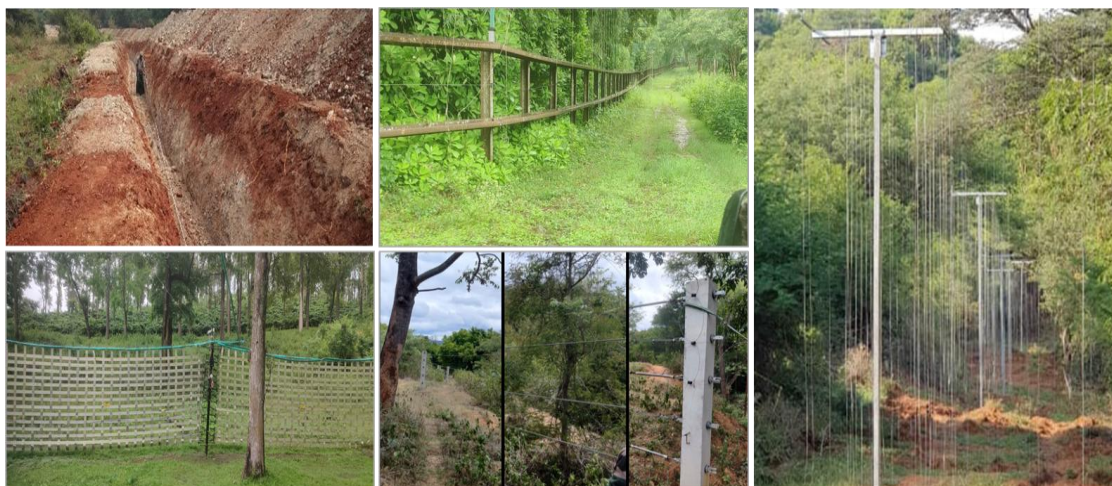
Fig-4.3: Types of Physical Barriers adopted in the Region (Top L to R) - Traditional EPT; Modern Fences- Rail Girder (KAR); Hanging Power Fence (All States); Steel Rope Fence (TN); AI-Smart Fence (KER)
